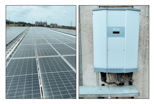
The project activity involves "Solar PV system" as the technology. The system is designed for a capacity of 998.64 KWp. The solar modules are mounted on module mounting structures of Al-Zn alloy coated steel on top of sheet roofs of the Berger paints manufacturing facility at Jejuri.
